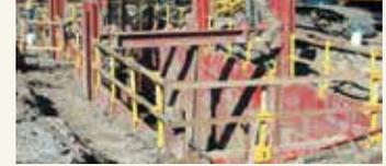
Pro-Tec Equipment's Railing Post System serves as an extra precautionary measure, providing temporary railing around excavations that involve trench shoring and shielding.
