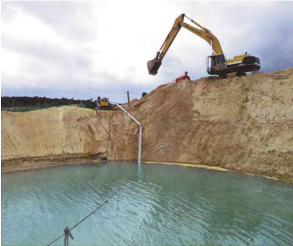
6" submersible pump driven by the HT6oDCV diesel power unit was used to divert ground water at a sand plant
