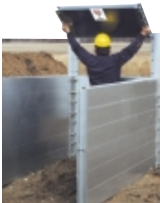
Modular Trench Shields
