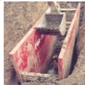
Steel Trench Shields
