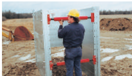
Adjustable spreaders pin securely in place to complete a 3-sided shield.
